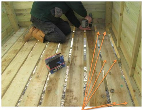
Evenly space out the 9 number 1.8m long 6x1 floor boards and fix down with 2 x 70mm screws at each floor bearer location
