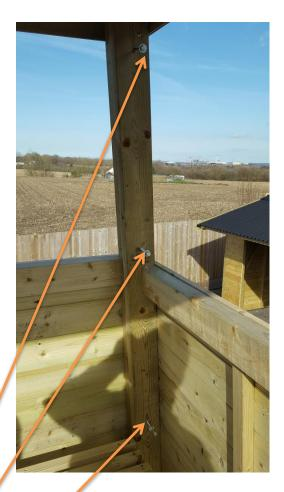
Pre-drill 6mm holes at the top middle and bottom (just above seat) of the 4 corners inside the blind and install M8 x 70mm coach screws and washers to secure the side panels to the front and back panels
