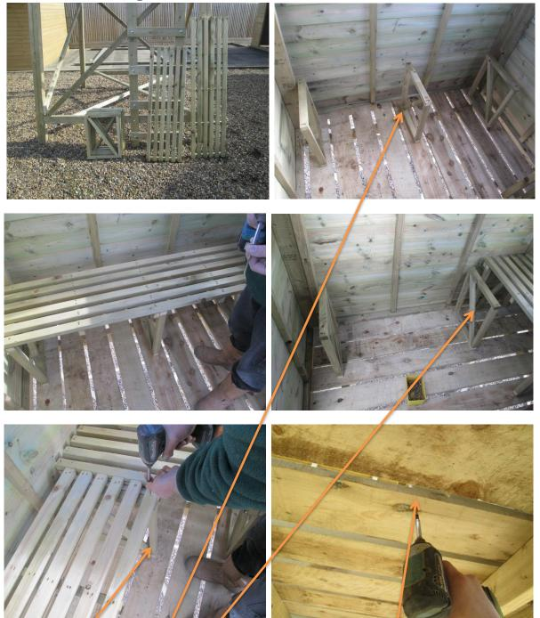
Evenly space out the 3 x long seat support frames, fit long seat to support legs and screw down to seat support frames using 2 x 70 nm screws for each seat support- pre drill holes using a 3mm drill bit prior to screwing to save splitting timber.
