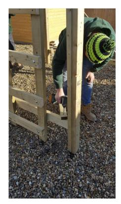
Remove the temporary 3.0m long 38x63mm diagonal brace fitted to aid lifting the blind to upright.
