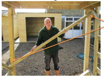
Fit the 2 number approx. 2.7m long 38x63mm side diagonal braces- ensure the braces are fitted apposing each other. Fitted on the inside of the support legs.
