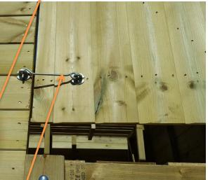
Fix the 2 x Tee hinges to the back of the blind door using 30mm screws.
