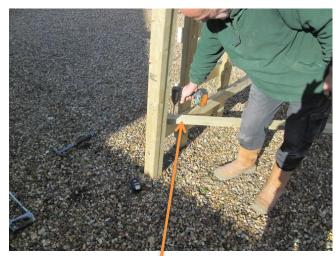
Fit the 2 number approx. 3.0m long 38x63mm bottom diagonal braces – note; one above bottom rails of front and back panel bottom 4x2 rails and one below. Use  $2 \times 100$ mm screws at each end of the braces to secure to the bottom rails of the front and back panels. Fit 4x4 brace support block at intersection of bottom diagonal braces using  $2 \times 100$ mm screws from above and  $2 \times 100$ mm screws from below.
