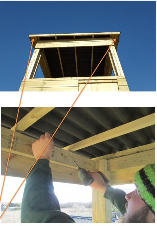
Ensure soffit boards are fitted at the sides not front and back- Square up roof before fixing down. Fix the roof panel to the blind framework using 2 x 70mm screw at each of the 6 roof purlin joint locations.
