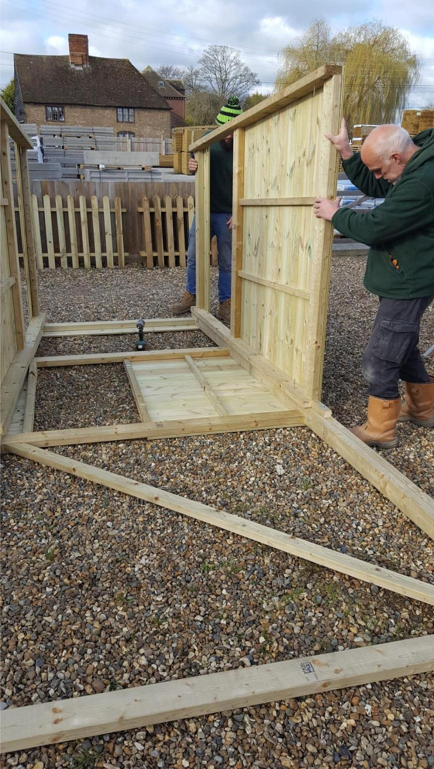
Fix second side panel as per previous side panel- fix using 3 x 100mm screws . These fixings are temporary.
