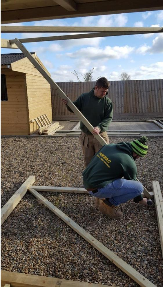
Temporarily fix one of the approx. 3.0m 38x63mm diagonal support braces between the bottom rails of the front and back frames for support whilst lifting the blind to upright using 1 x 100mm screw at each end
