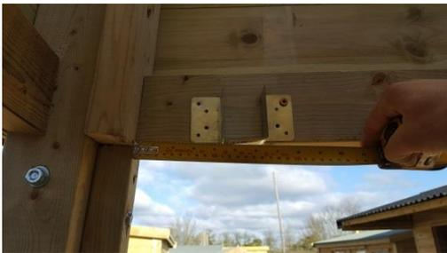
Fit the floor bearer joist hangers to the bottom rail of the side panels using 30mm screws provided. **Must be on the short side panels**
