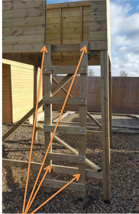
Fit ladder to front panel doorway. Fix ladder to top and bottom rails using 4 X M10 x 110mm coach bolts , washers and nuts. Pre-drill holes using 10mm drill bit. 4 x 110mm coach bolts, washers and nuts needed.
