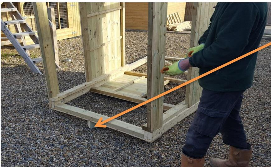
Lift the blind and temporarily fit the 4x4 diagonal brace support block under the blind to aid lifting the blind to upright
