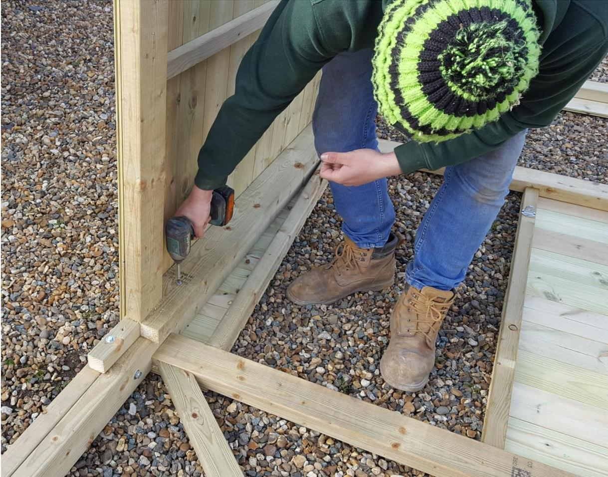
Fix first side panel to front panel using 100mm screws provided- top middle and bottom, these fixings are temporary fixings. ( 3 x 100mm screws needed)
