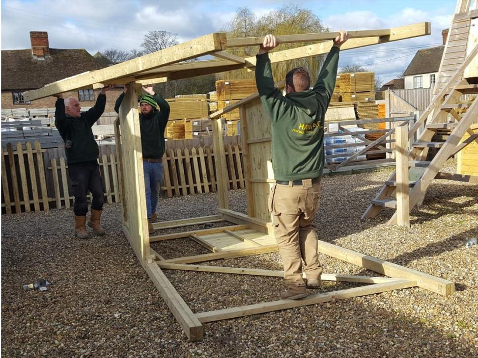
Carefully lift back panel section onto side panels and fix as before using 3 x 100mm screws to side walls.
