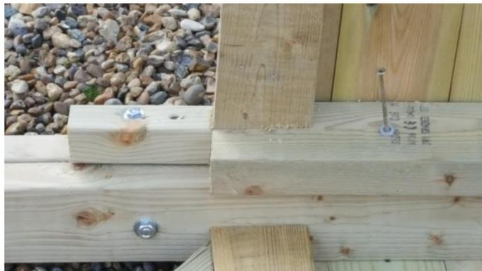
Fit first side panel to top of main support leg ensuring the side wall is fitted tight to the support block of the main frame
