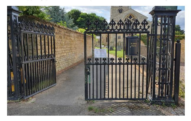
There is no requirement for any welding or drilling of the gate metalwork. The post box attaches via a simple clamp plate. The existing fabric of the gate will not be affected in anyway.
