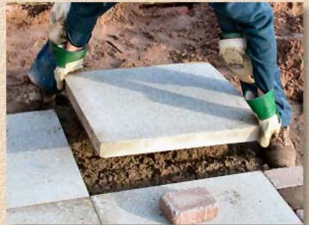
Lifting a small flag into place
