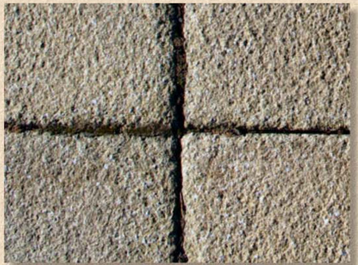
Close Joint - flags have narrow 1-3mm joint
