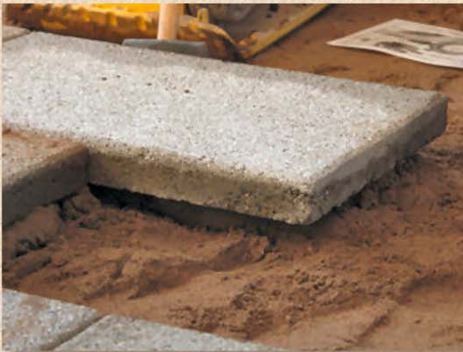
You don't need a degree in engineering to see that this type of construction offers buggerrall in the way of support for flagstones
