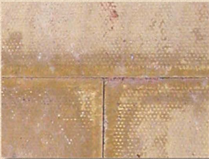
Butt Joint - flags in direct contact
