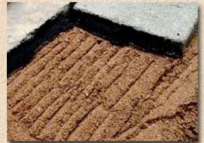
Mortar is battered onto receiving edges
