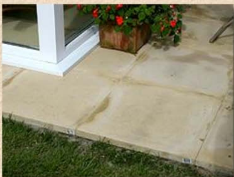
Flags laid to a free edge in a garden setting
