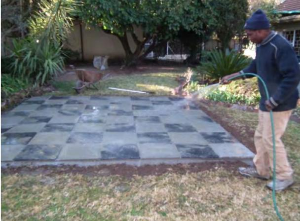
Water again. It is very important to keep the cement wet to prevent cracking at least for a couple of days.
