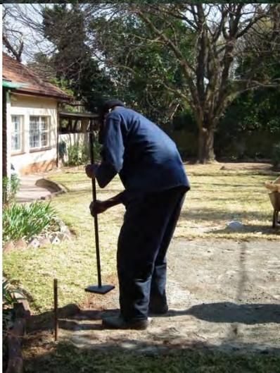
Now compacting the sub-base with sand/cement sealing layer is recommended. This can be done with a tamper (as in the picture) or better is a compactor.
