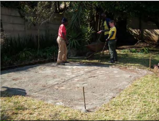
Sub-base preparation is very important for the final result. You don't want grass or weeds to be able to grow between the slabs and you want the slabs to remain in place with use. If there is a chance that vehicle will drive onto the slabs extra care needs to be taken to make sure the slabs are well set and the sub-base is well compacted.
