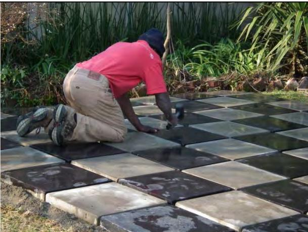
Then with a rubber mallet, again, tap the slabs so they are all at the same level with the even 10 mm spacing for the grout.
