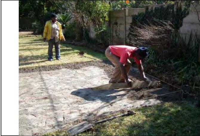
Spread using a flat piece of wood and use a level to make sure flat, level and smooth.
