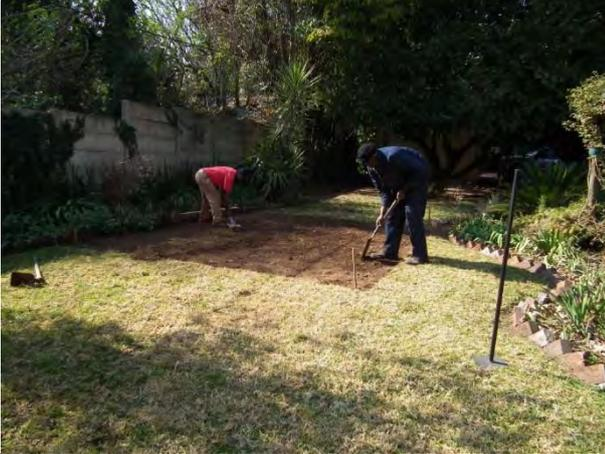
Having exposed a good sub-base now you need to get it level. Using a long plank and spirit level get the base as level as possible.
