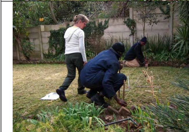
Mark out your area roughly 4 x 4 metres with a straight line using string and pegs.
