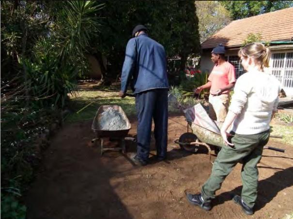
Make a dry riversand (coarse) and cement mix roughly four parts sand to one part cement.
