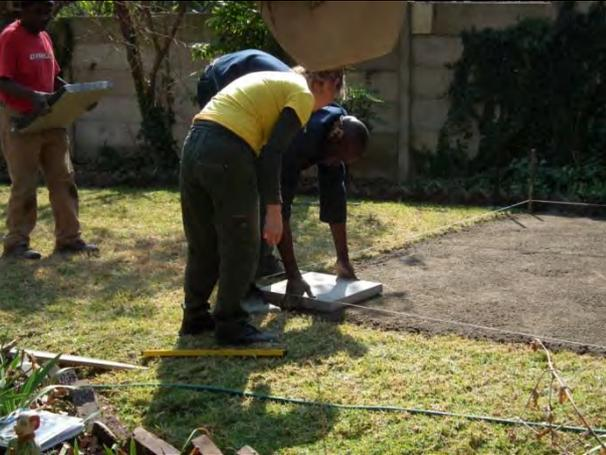
Do your line with level and string then start laying your slabs with a 10 mm gap in between each slab for the grouting.
