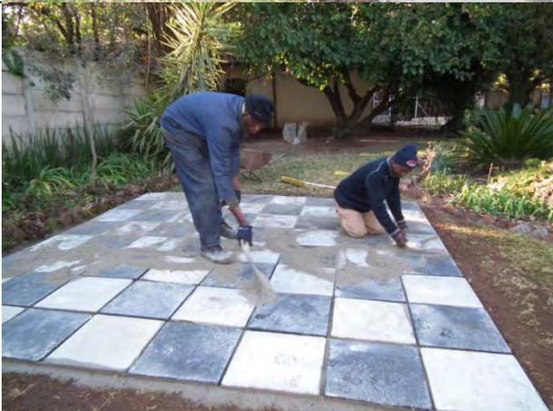
Leave overnight and the next day you then spread a dry cement mix over the board making sure that all the gaps are full of the mixture.
