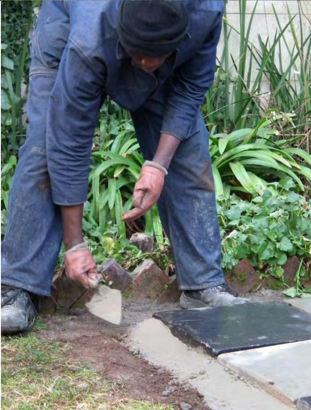
Make a nice edge using cement or you can use tiles. This to support the edges of the slabs so that they can't move out of place.
