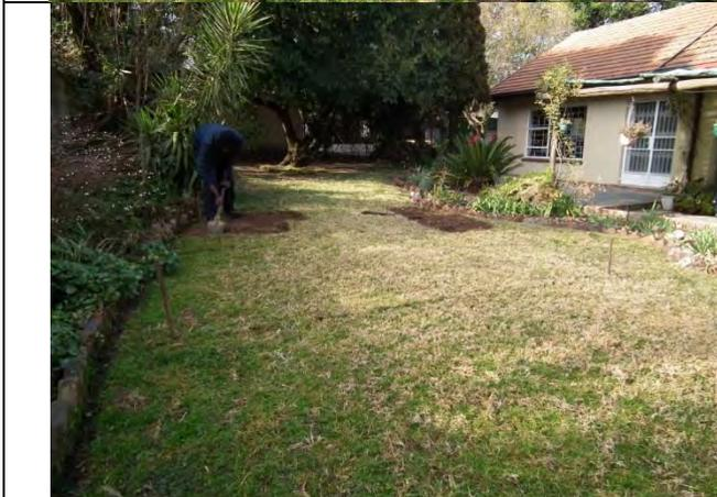
Now you need to remove any grass or organic materials that could rot over time and could cause the slabs to subside over time.
