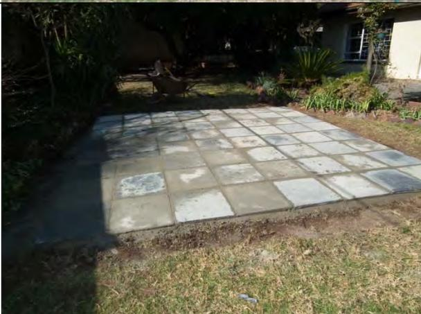
When the slabs have settled (typically the next morning) you can use a stiff brush or broom to brush off the excess cement/sand.
