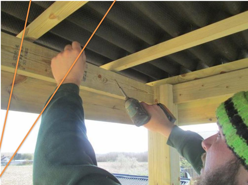
Ensure soffit boards are fitted at the sides not front and back- Square up roof before fixing down. Fix the roof panel to the blind framework using 2 x 70mm screw at each of the 6 roof purlin joint locations.
