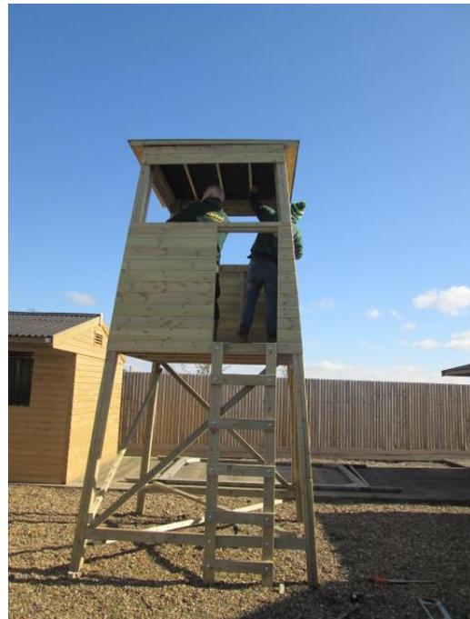
Carefully lift roof panel onto top of blind
