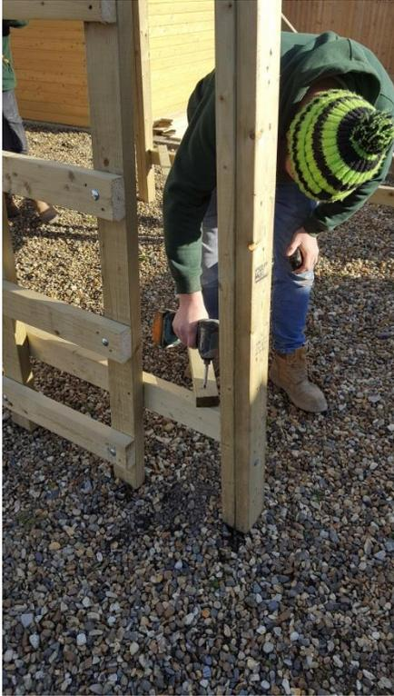
Remove the temporary 3.0m long 38x63mm diagonal brace fitted to aid lifting the blind to upright.
