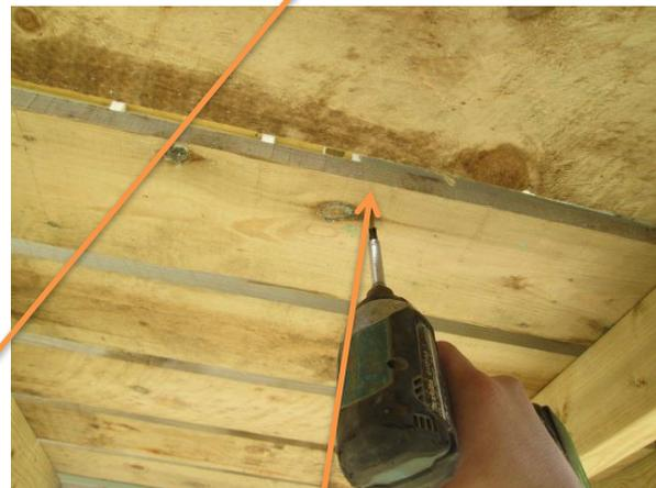
Evenly space out the 3 x long seat support frames, fit long seat to support legs and screw down to seat support frames using 2 x 70mm screws for each seat support- pre drill holes using a 3mm drill bit prior to screwing to save splitting timber.
