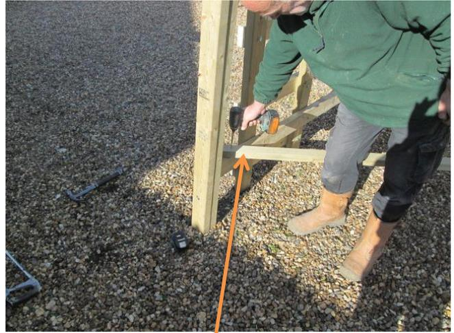
Fit the 2 number approx. 3.0m long 38x63mm bottom diagonal braces – note; one above bottom rails of front and back panel bottom 4x2 rails and one below. Use 2 x 100mm screws at each end of the braces to secure to the bottom rails of the front and back panels. Fit 4x4 brace support block at intersection of bottom diagonal braces using 2 x 100mm screws from above and 2 x 100mm screws from below.
