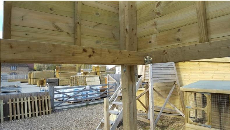
Fit the 3 number 4x2 floor bearers to the hangers and screw fix to secure using 30mm screws provided.
