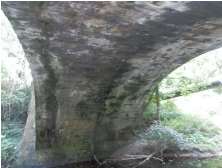
The older, downstream side on the left, newer upstream side on the right.
