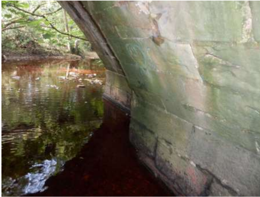
The upstream arch, in the background, is slightly wider.
