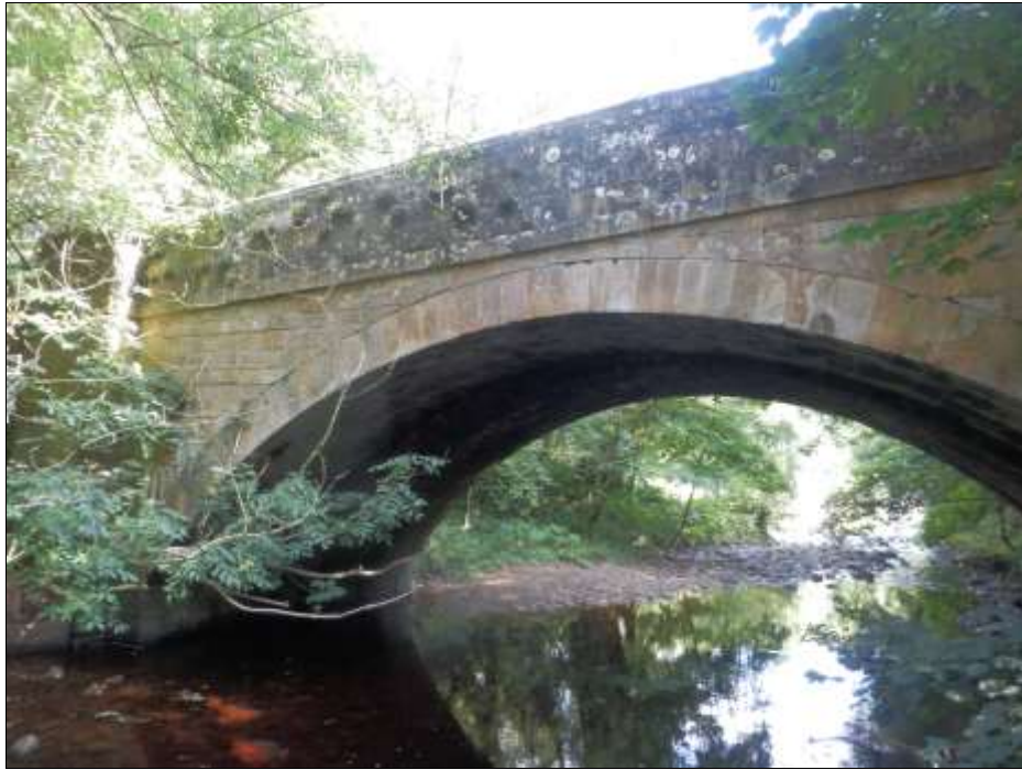
The single arch on the upstream side
