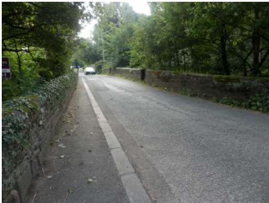
The narrow downstream pavement and the upstream pedestrian refuges.
