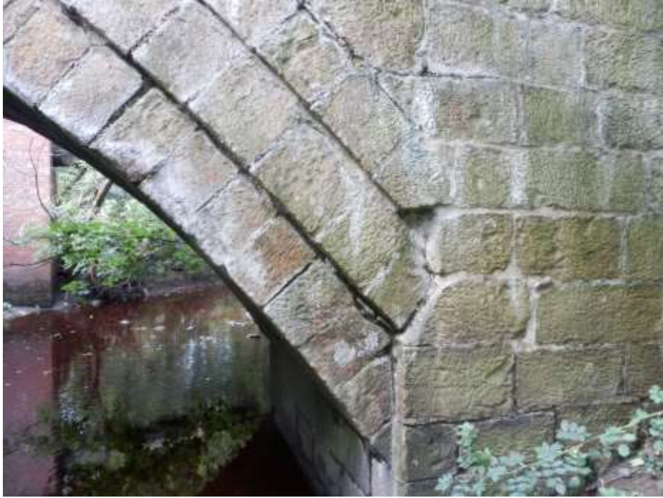
The triple arch on the downstream side.
