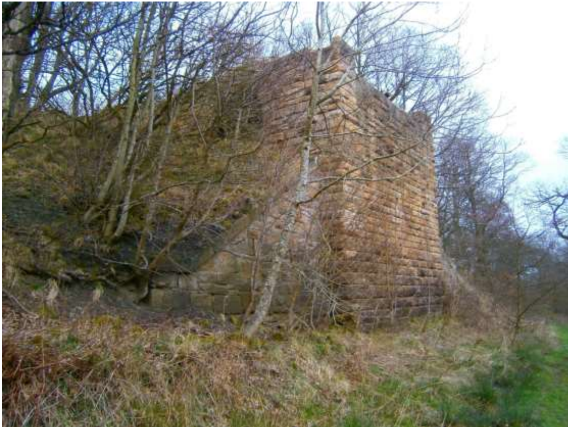
The abutments on the north (Lartington) side.
