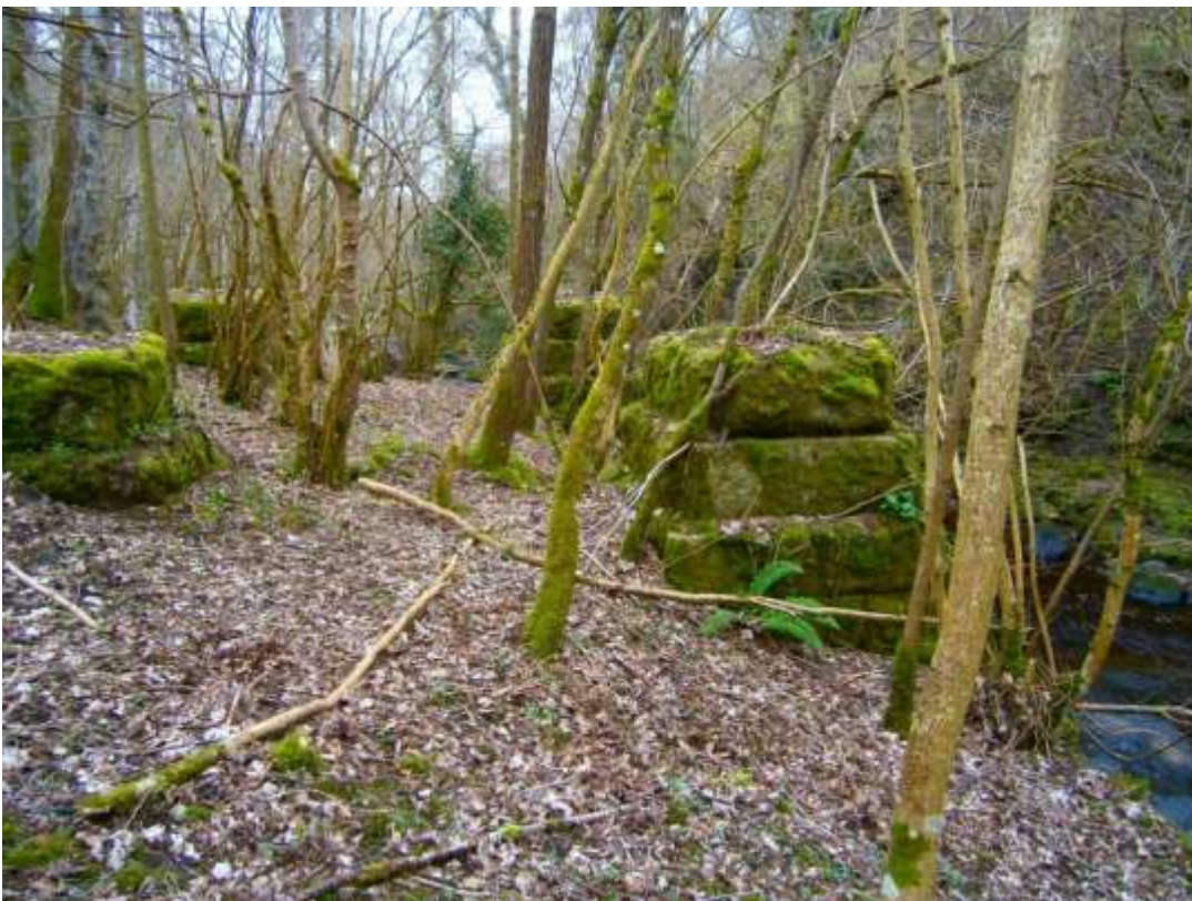
The stone foundations of the piers on the north bank.
