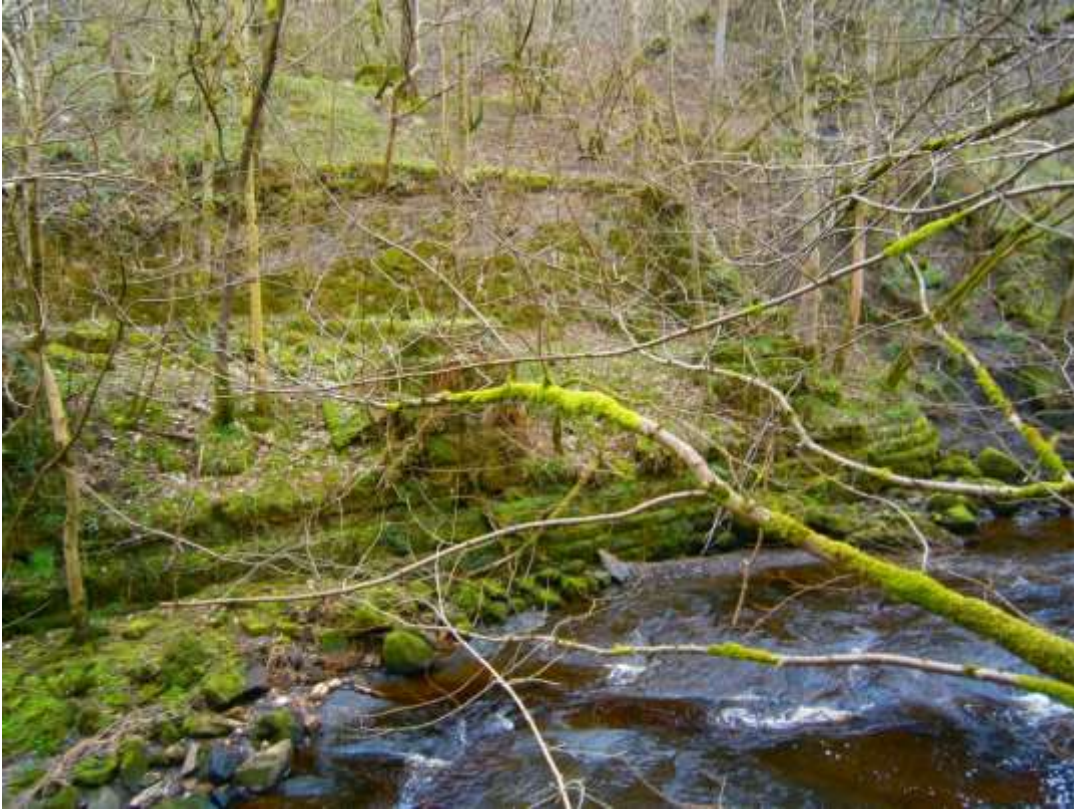
The south abutments.
