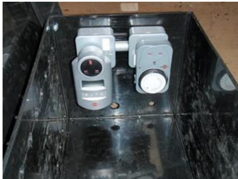
It is not possible to plug two timers into a standard double socket so for this reason multiple single sockets are required. To accommodate the timers the sockets must be spaced at least 50mm apart.
