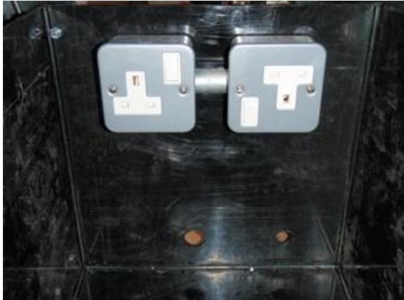
Both the air blower and solenoid valve require timers; the timer is plugged into the socket and the device is plugged into the timer.
