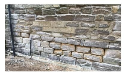
The above photo shows some new facing stones that have been fitted. Part of the adjacent pointing had to be removed and will be replaced with lime mortar. The cement used previously retains water in the walls and encourages deterioration of stone.
