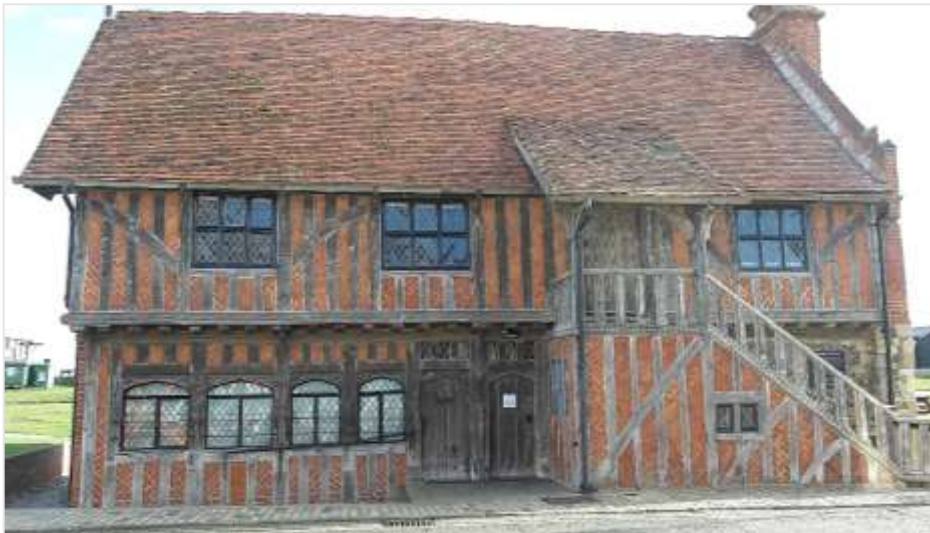
Figure 4 View of the Moot Hall from West.
