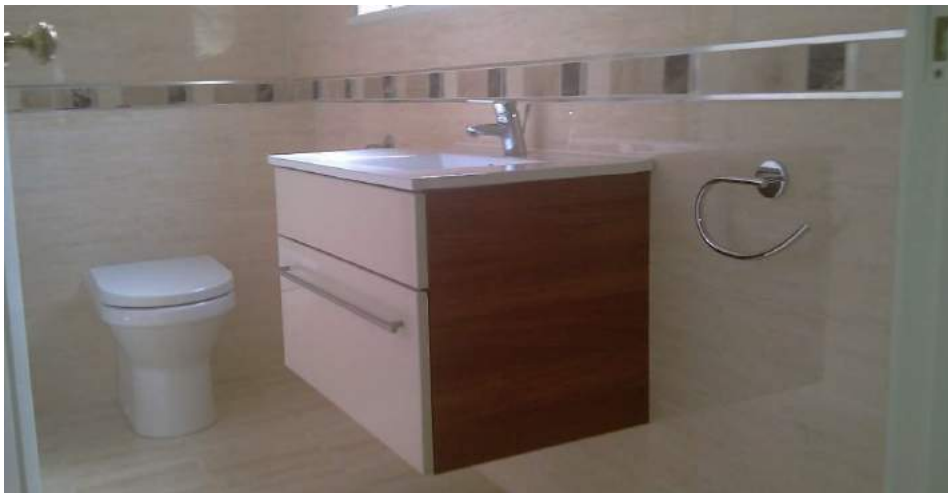
Bathroom Renovations // Page Twelve
