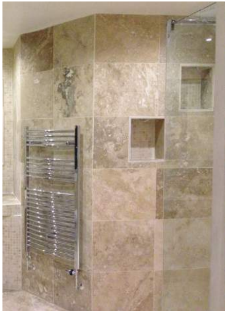
Bathroom Renovations // Page Two
