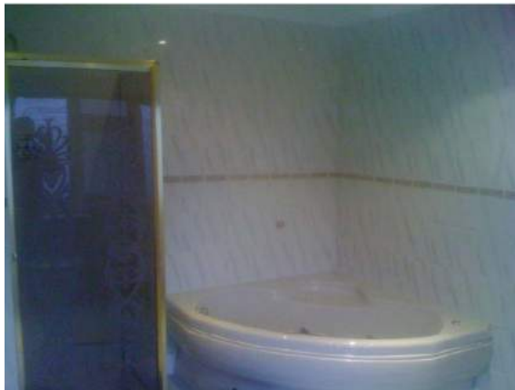
Bathroom Renovations // Page Six
