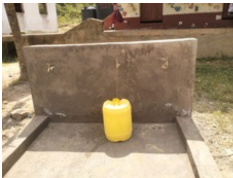
New taps fitted to the water station
