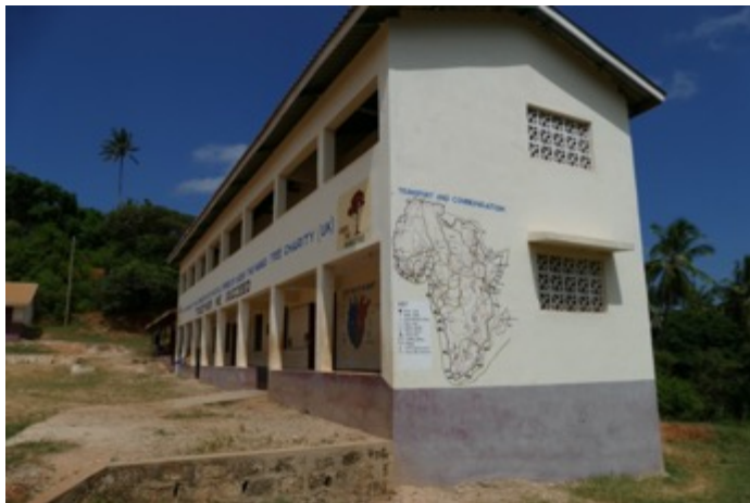
Photo of the four roomed classroom, funded by UTMT, in 2018
