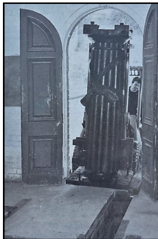
Inspecting the new floor to receive the engine and manoeuvring the massive central column through the narrow doors
